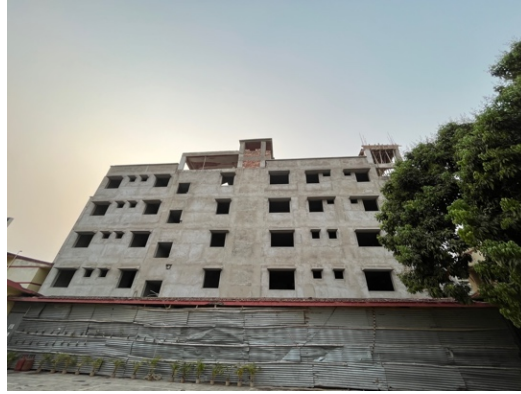
The construction in February 2023
