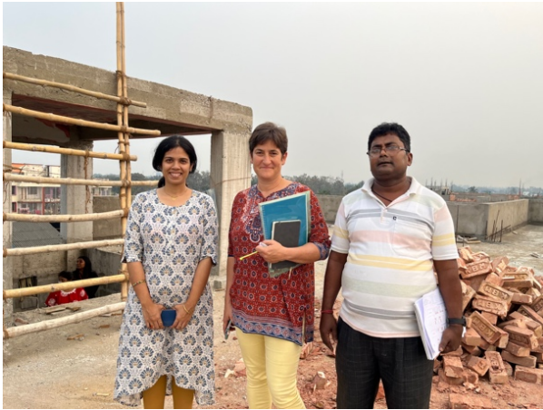
On the roof of the building with Bashwati Roy and Nishi Kanta Nayak from WIF. A roof garden for the senior citizens is to be built here.
